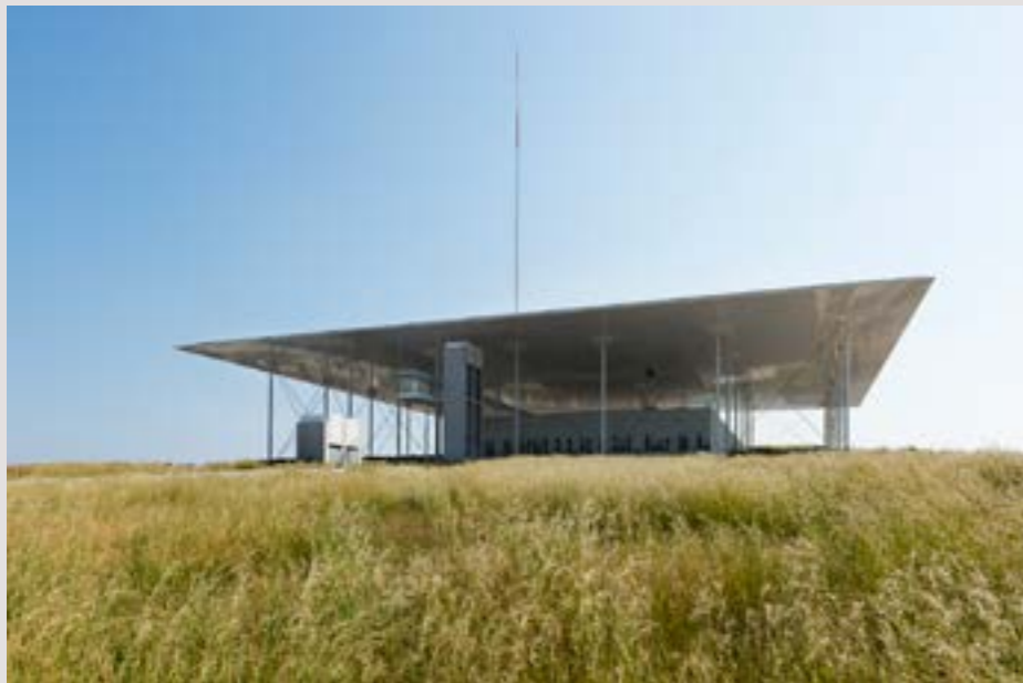
[←] General view of the canopy. SNFCC, Photographer: Y. YeroLymbos
